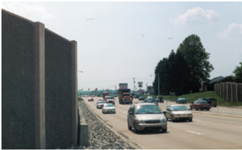
Traffic noise wall along a roadway
