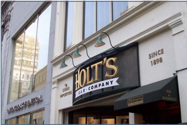
Gooseneck lighting in Philadelphia, Pennsylvania
