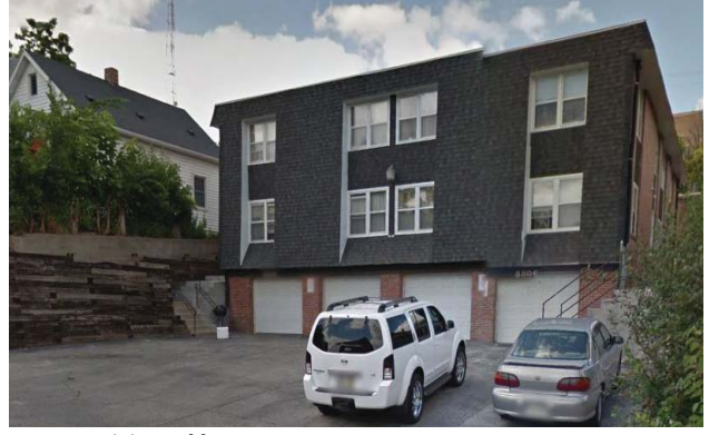
Incompatible roof forms
