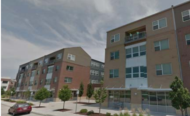
Charge in material at upper level
