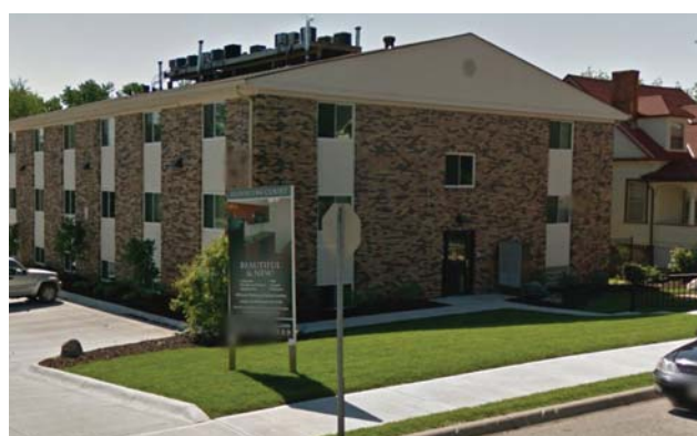
No transitional element at building entrance
