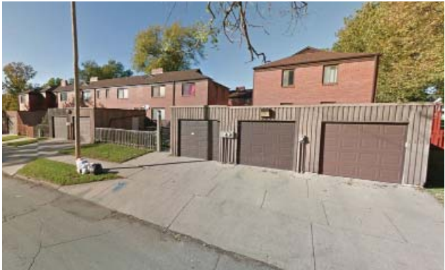
Garages with no pedestrian entrance facing the street
