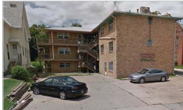
No transitional element at building entrance
