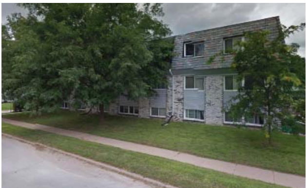
No entrance element facing the street
