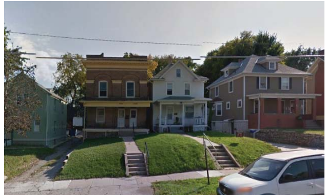
Incompatible roof forms
