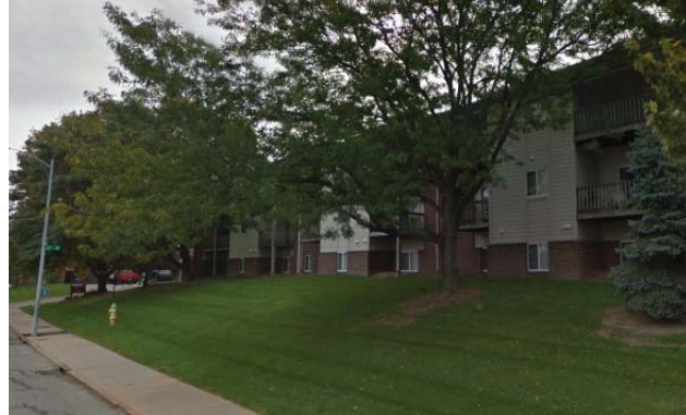
No entrance element facing the street
