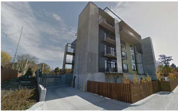
Structured parking below grade
