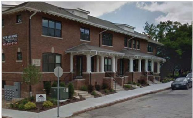
Elevated stoop and canopy at building entrances
