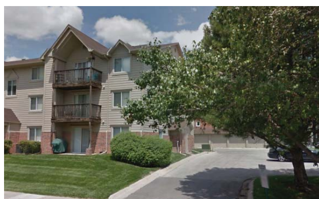
Garage structure at rear
