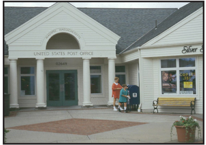
Post Office and Shops, Mashpee Commons, Mashpee, MA
