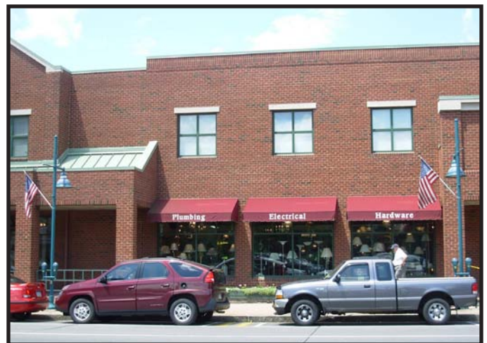
Articulated Facade with Awnings, Rolliers, Mount Lebanon
