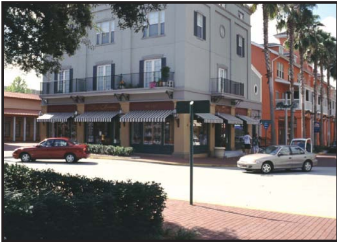
Offices Over First Floor Retail, Celebration, FL
