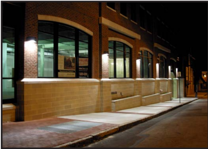
Wall Pack Lights that illuminate sidewalk and prevent upward glare
