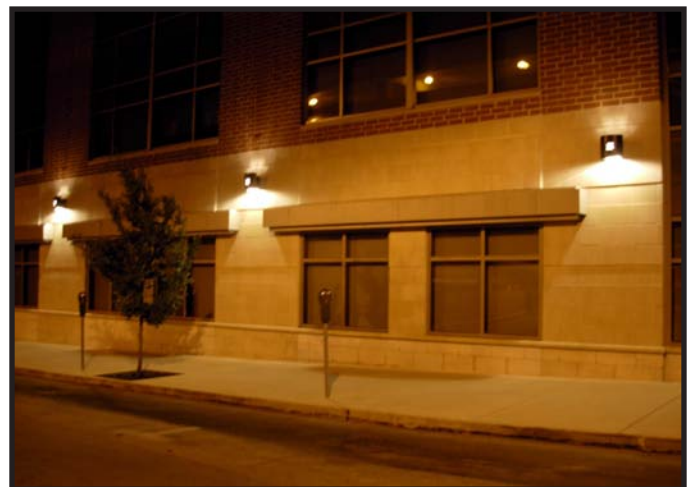
Lighting Packs with Glare Shields
