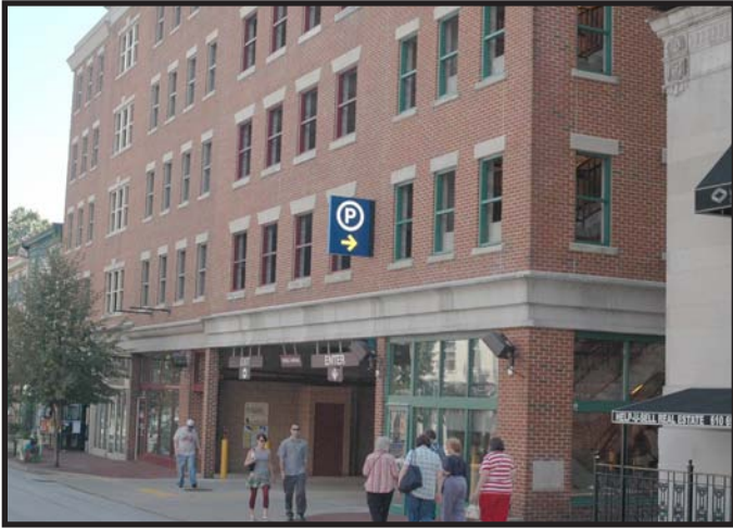
West Chester deck parking structure with an architectural character consistent with nearby buildings.
