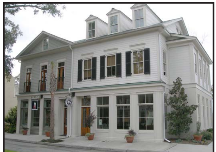
Live Work Units, Habersham - SC
