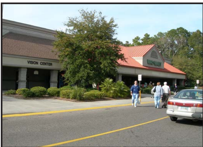
Walmart with Roof Projection & Portico, Hilton Head, SC
