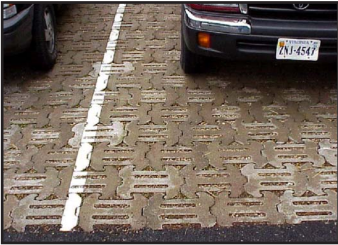
Unit Pavers as Porus Pavement
