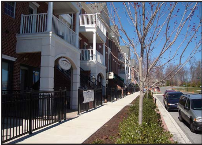
Live-Work Units, Eagleview - Lionville, PA
