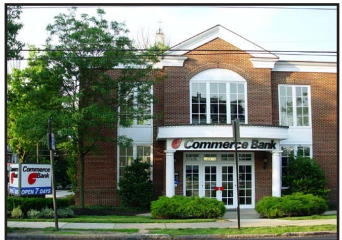
New Commerce Bank with Portico, Media, PA
