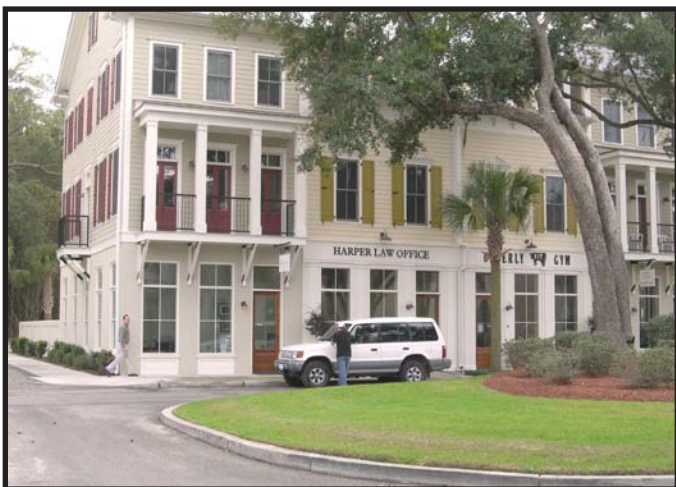
Live Work Units, Habersham - SC
