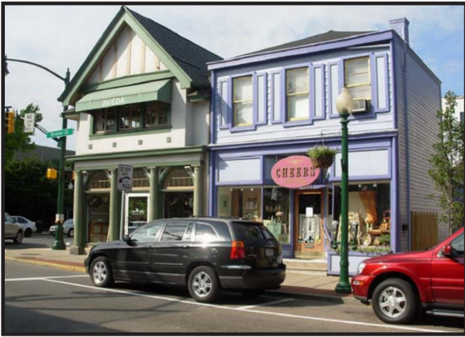
Two-story Building, Sewickley, PA
