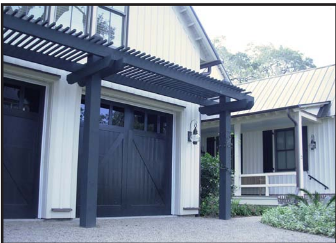
Detached Garage off Alley, Palmetto Bluff, Bluffton, SC
