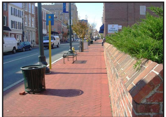
Off-Street Parking Screened by Brick Wall, West Chester, PA
