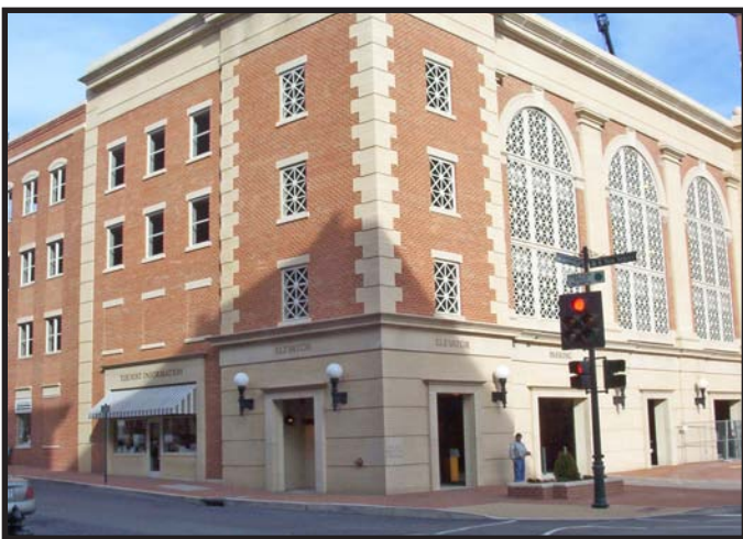
Deck Parking Structure, Staunton, VA
