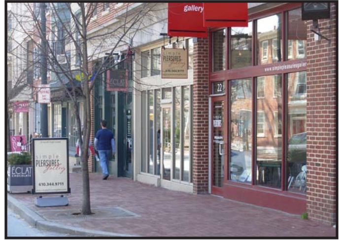
Liner shops of the West Chester deck parking structure.
