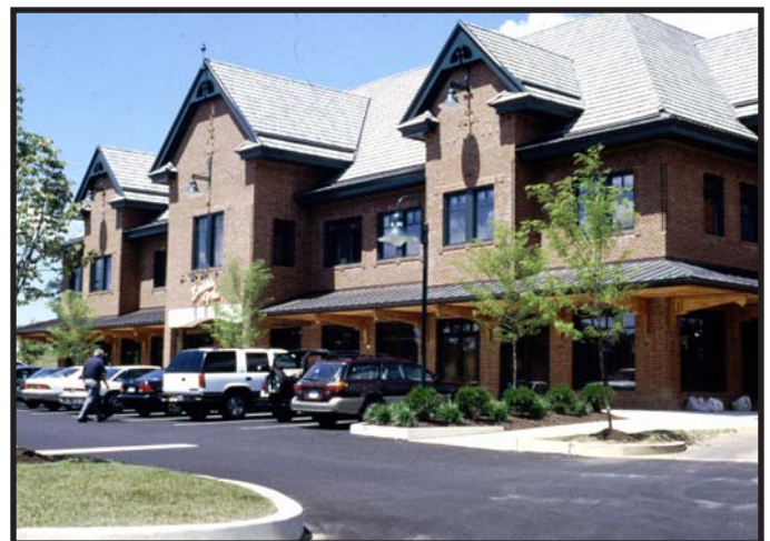
Ground Floor Restaurant and Second Floor Offices & Retail: Egelview Town Center, PA
