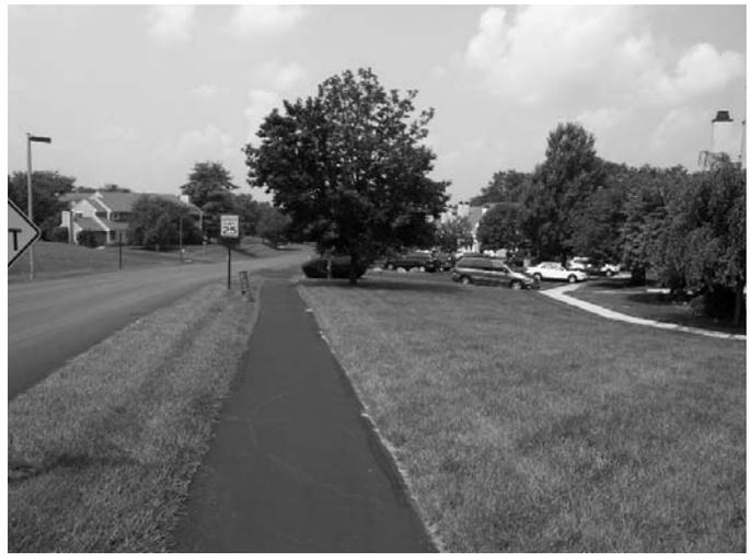
Macadam is preferred for paths since it has lower maintenance cost and is less susceptible to stormwater erosion.
