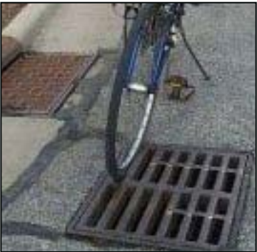
Dangerous Drainage Grate Condition; this example is dangerous due to the grate running parallel to the roadway, creating a trap for bicycle tires.
