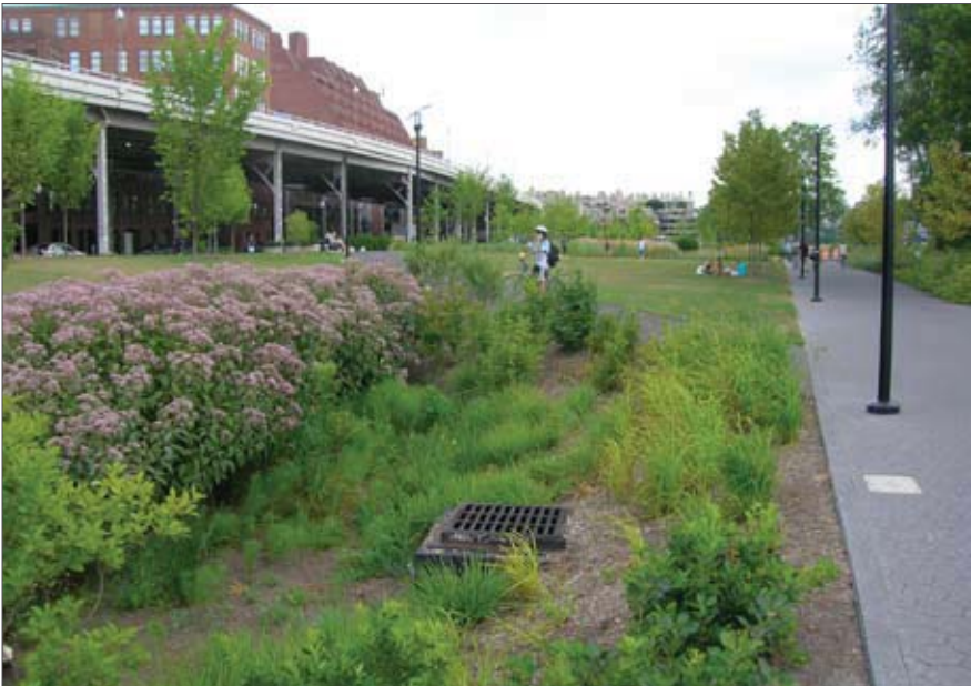
Landscaping used on the Capital Crescent Trail, Washington DC, shows how stormwater treatment can be tied to aesthetically pleasing plantings.
