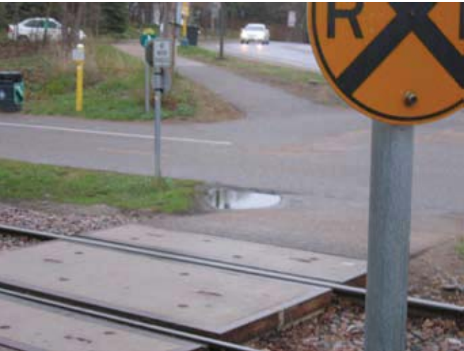
The “flangeway filler” eliminates the gap in the path of travel for pedestrians crossing railroad tracks. The filler, consisting of a rubber insert, will deflect downward with the weight of a train and does not affect railway function.
