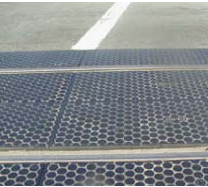
Installing a rubber surface rather than asphalt around railroad flangeways reduces changes in level and other maintenance problems.
