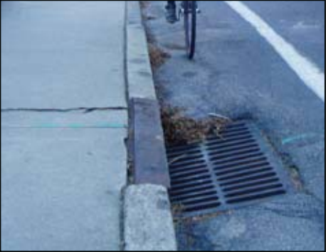
Dangerous Drainage Grate Condition; this example is dangerous due to the surrounding paving condition (when the road was resurfaced the drainage grate remained at the same height).
