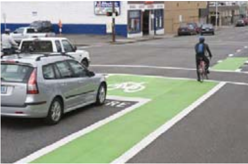
Above and below: Bike boxes filled in with color to emphasize allocation of space to bicycle traffic.
