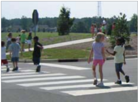
A variety of patterns are possible in designing a crosswalk; an example of a 'continental' design is shown above.
