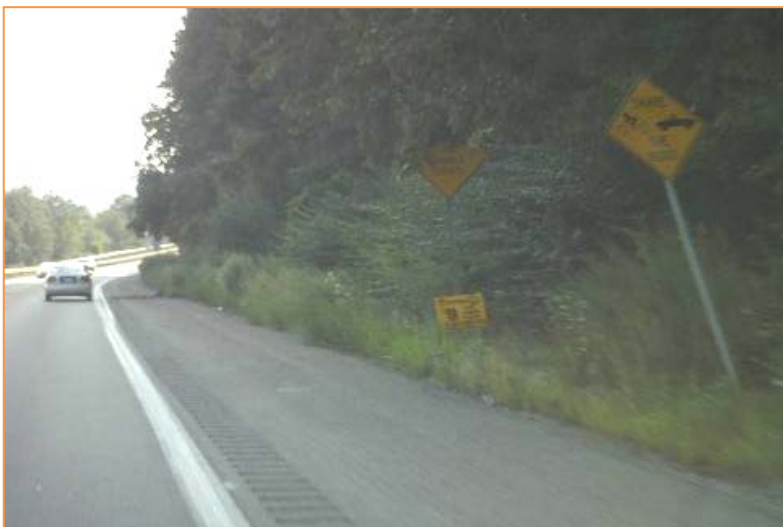
Rumble Strips on SR 837 in West Mifflin
