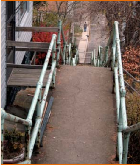
Public Steps and Pedestrian, South Side Slopes Photo: Lynn Heckman
