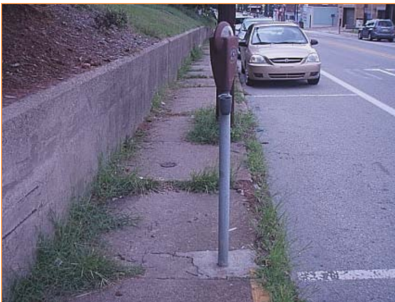
Sidewalk clear width in Blawnox is reduced by utilities and parking meters. Maintenance is needed for some sections.
