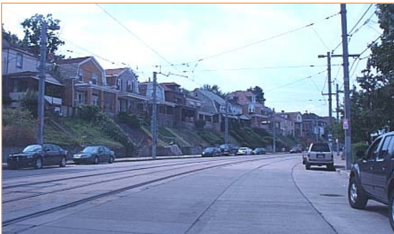
Broadway Avenue has ample capacity for accommodating bike lane
