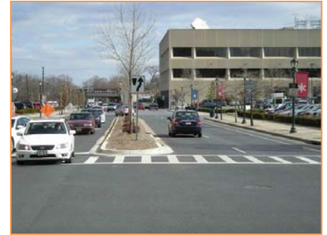
Suburban roadway with high visibility crosswalks, median and bike lanes
